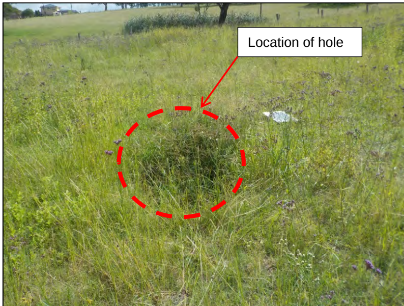
Figure 6: Hole observed at surface of neighbouring property. The hole diameter was approximately 2 m. The location of the hole coincides with the approximate location of the “Tunnel Mouth” as shown on RT603
